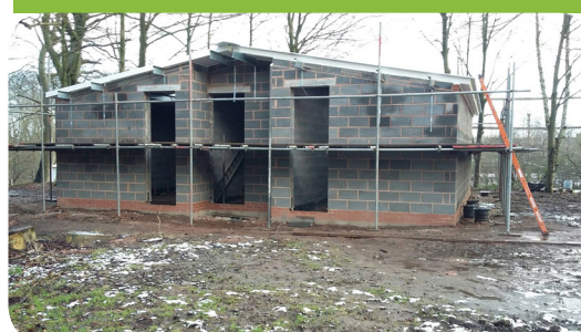
Day Block under construction
